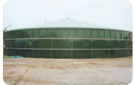
Figure 1. Slurry store fitted with a rigid cover
